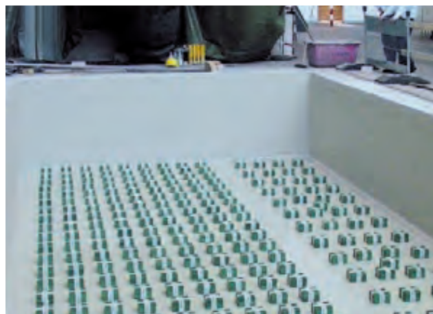
Foundation pit with Bilz insulation pads laid out
